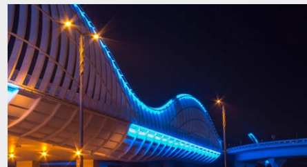
Architectural outdoor lighting
